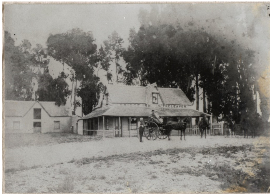
Exterior of the Belfast Bridge Inn, with the owner Mr Samuel Treleaven serving a customer (1870's). Source: https://canterburystories.nz/collections/community/bdmt/local-scenes-and-places/ccl-cs-80524
