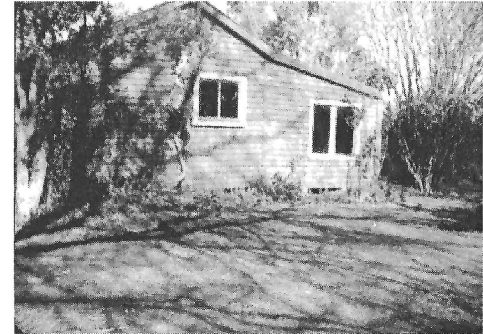
Cottage at 663 Main North Road
